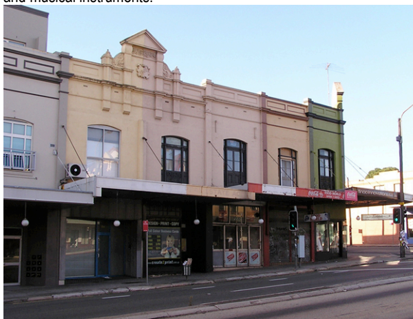
Figure 5.23 and 5.24. The original balcony to the upper level of this group has been removed although evidence can still be seen through the original door openings and in the shadow lines in the rendered facade
