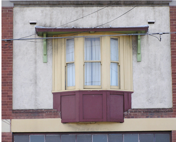
Figure 5.19 an original boxed bay window
