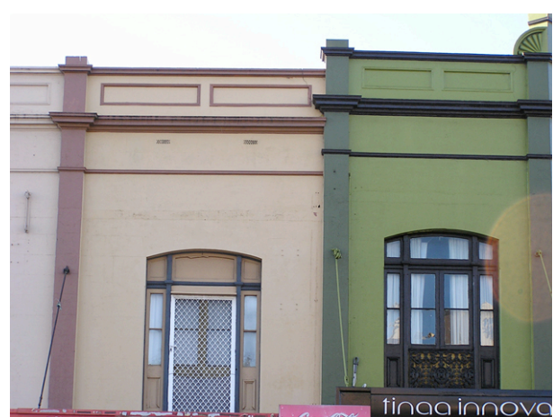
Figure 5.23 and 5.24. The original balcony to the upper level of this group has been removed although evidence can still be seen through the original door openings and in the shadow lines in the rendered facade
