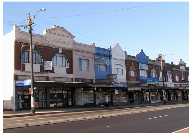
Figure 5.18. This group also demonstrates a strong parapet line with the modulation of the different bays creating a visually interesting skyline. Remnants of the original arched veranda openings to the upstairs residence can still be seen although all have been infilled over the years.
