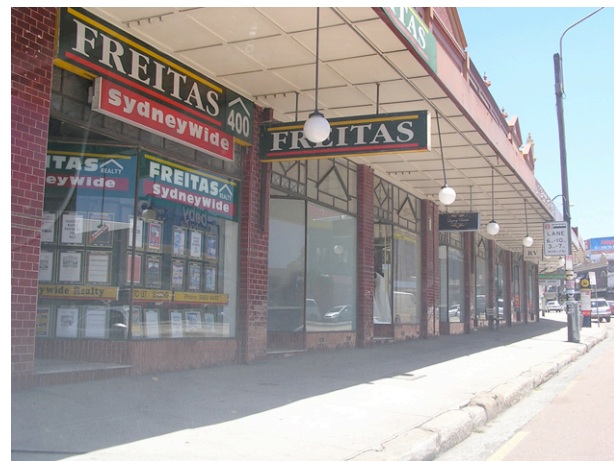
Figure 5.22. This group of shopfronts has been repaired and reinstated as part of a redevelopment of the remainder of the site. The glazed ceramic tiles are typical of the late Federation – Inter-War shopfront.
