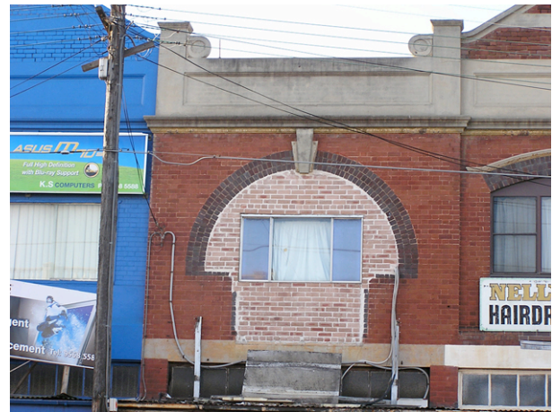
Figure 5.20. This arched veranda opening has been infilled crudely but the original brickwork is intact and has not been rendered or painted, making the layer readily reversible.
